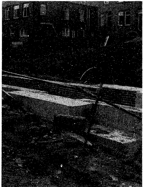
Completed brick facing to the main chamber walls of Lock 37E behind Marsden Band Club.
